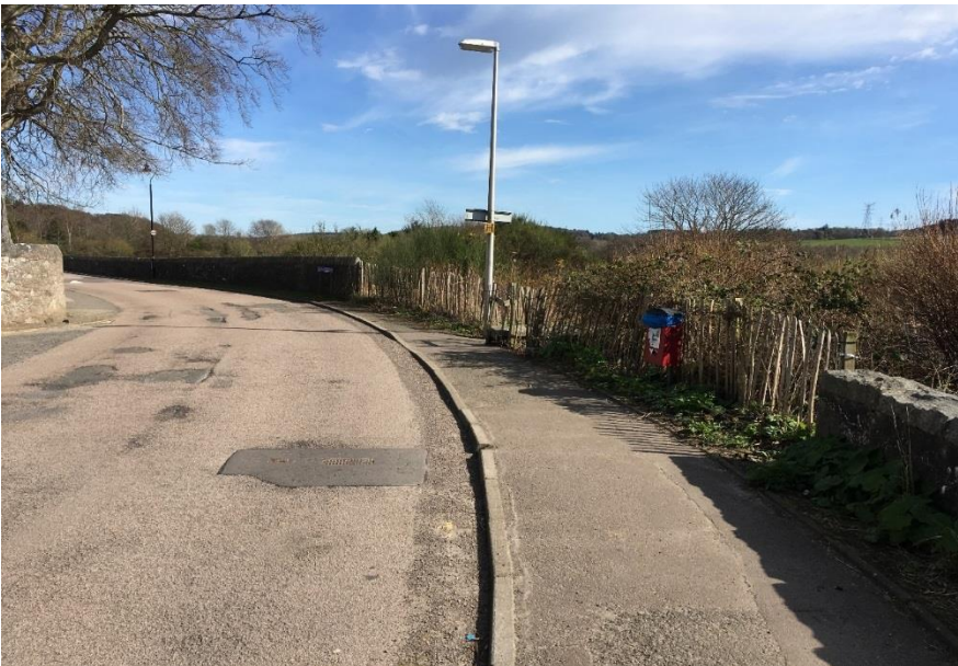
Figure 9: Vicinity around old Morison's Bridge entrance
