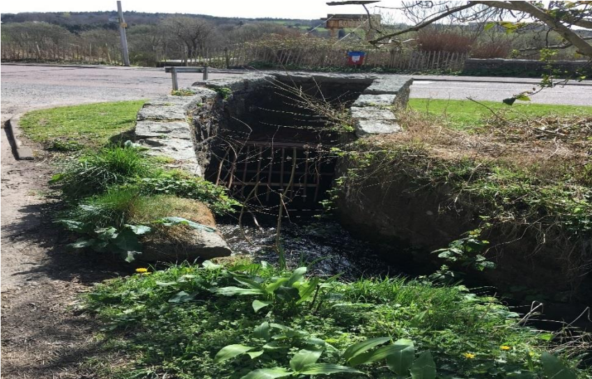
Figure 6: Burn of Cults Culvert Inlet
